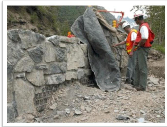
A retaining wall along Going-to-the-Sun Road is reinforced and a replica stone veneer makes it blend with the original design
