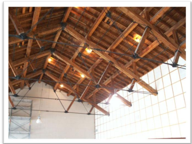
Many Glacier Hotel dining room ceiling during restoration
